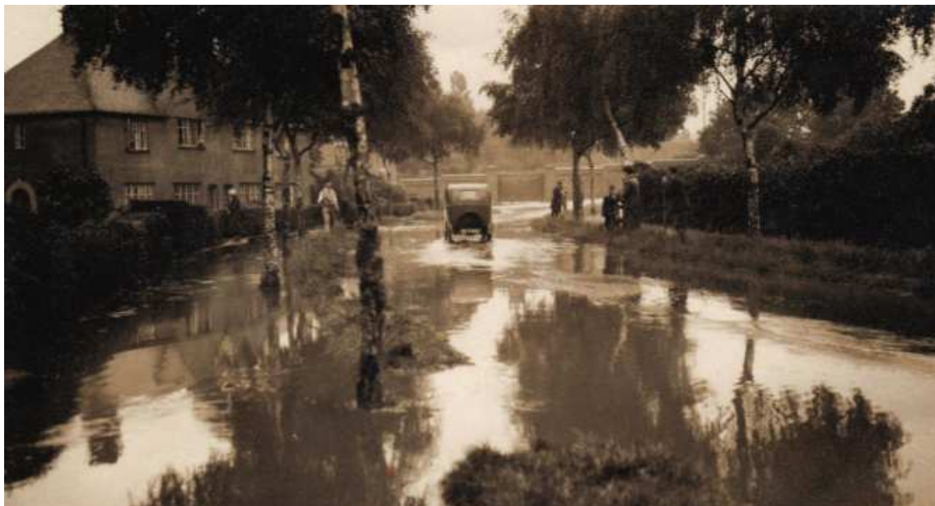
Flooding in Margaret Grove, June 1931 (above) and more recently in 2005 in the Valley Site (below and over)
