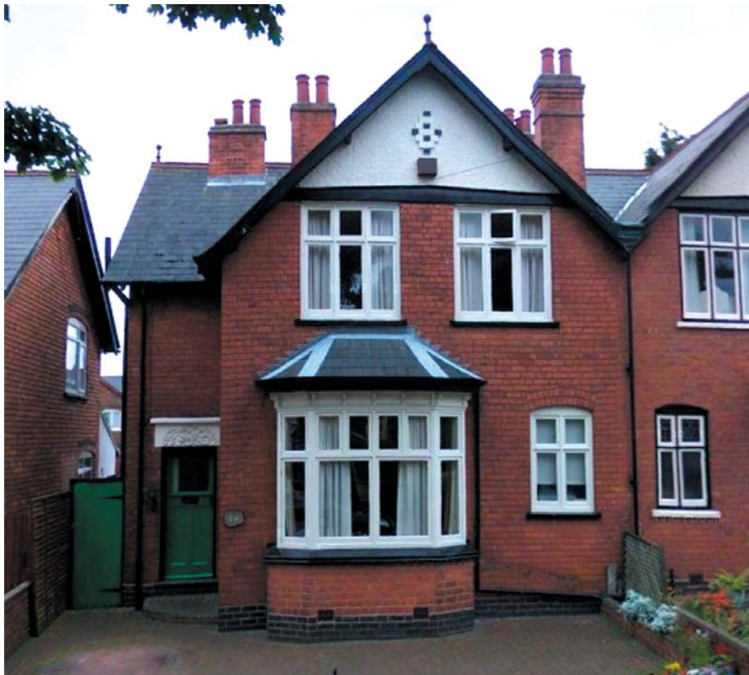
▼ Ideal Village - House with original windows and door intact
