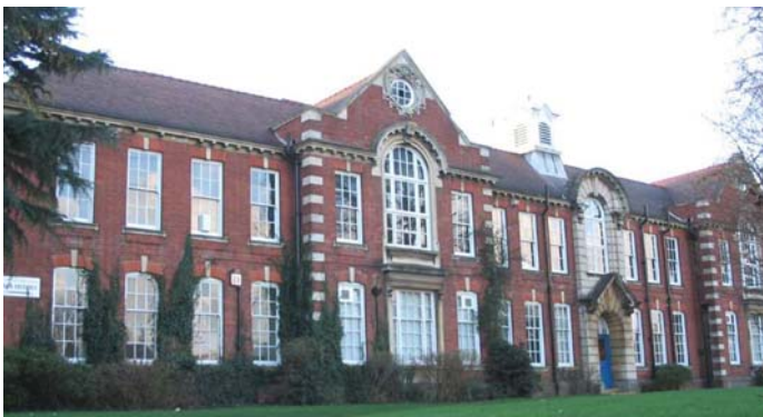
▲ Bromsgrove's Parkside School was built 1909-1912 to the design of A.Vernon Rowe
